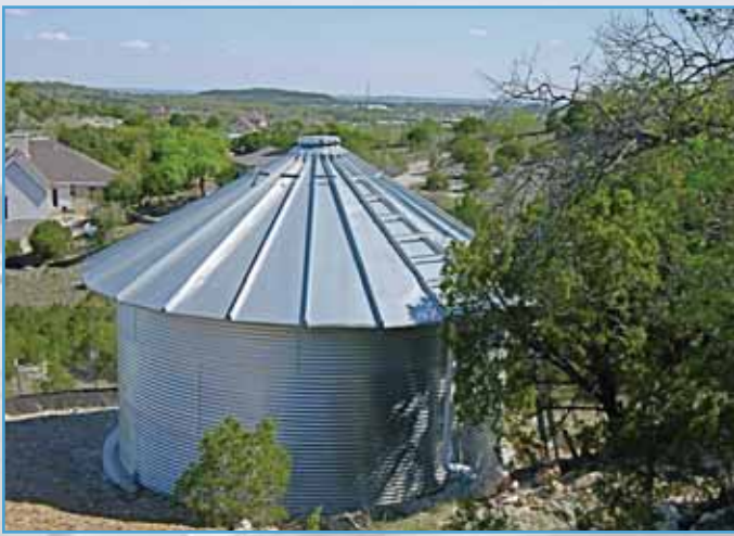
Water Storage Tank for agricultural use
