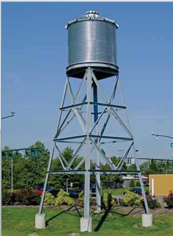
Overhead Water Tank mounted on tower
