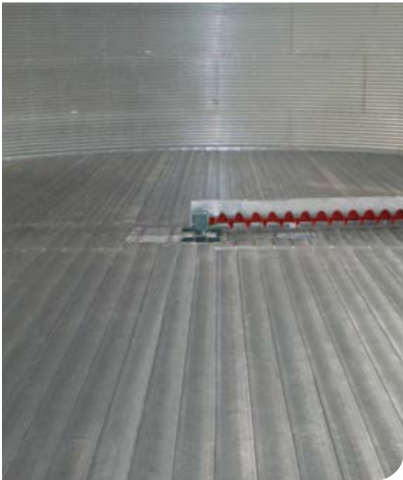
Full perforated plank floors allow for drying or conditioning air to distribute evenly up through the stored product.
