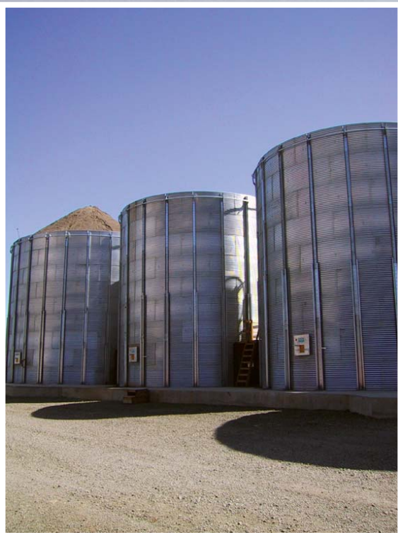
Aggregate Silos with open tops are easy to fill using a portable inclined conveyor.
