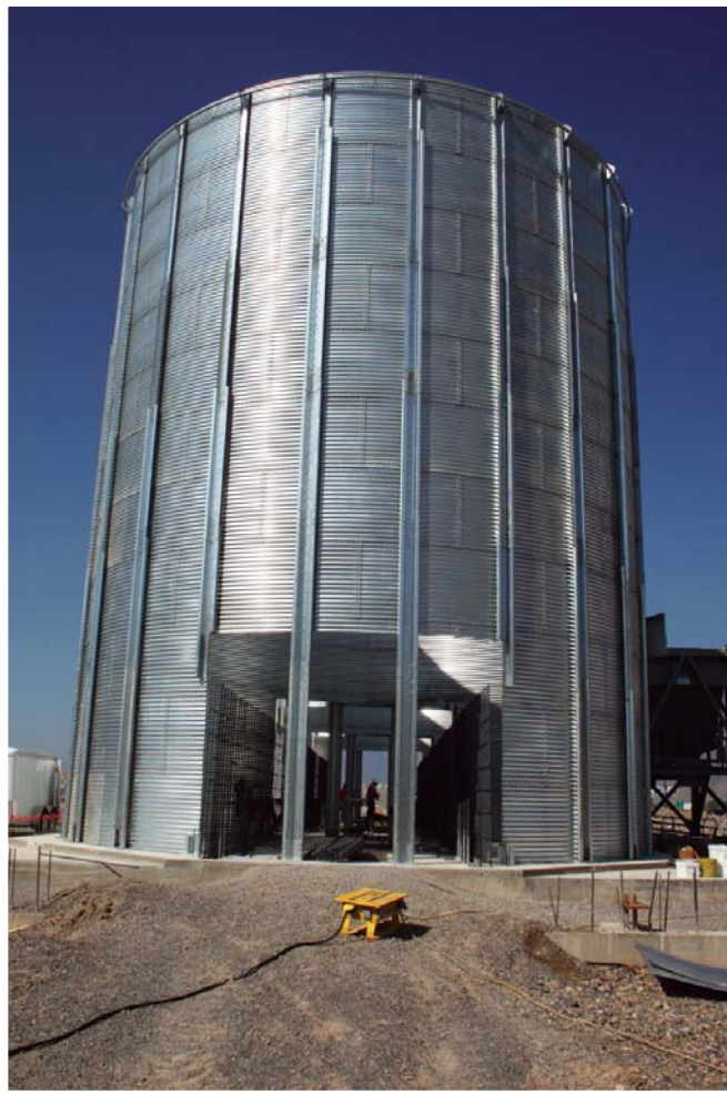
Aggregate Silos are manufactured from heavy gauge stiffeners and 8 gauge wall sheets.
