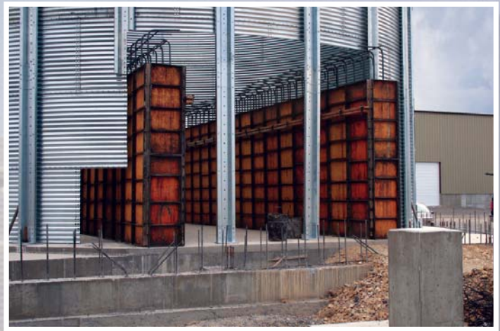
Concrete forms for the tunnel enclosing the reclaim conveyor.
