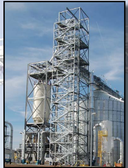
20' x 20' x 136' (6.10 m x 6.10 m x 41.45 m) Structural tower with self supporting switch-back stairway.
