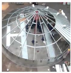
Lower roof panels are bolted to clips at the eave and fastened to the roof transition strip with self-drilling fasteners. Panels bolt together at the roof ribs.
