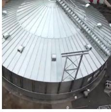
Catwalk supports, if present, can now be attached to the external stiffeners on the silo wall. Silo wall and assembled roof are raised one ring at a time (1.08 m/3.5 ft per lift) with hydraulic jacks.
