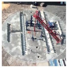
Silo erection stairway attaches to the jinn pole and rotates around the floor area to assist in roof structure and roof panel installation.
