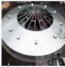
Upper roof panels bolt to clips at the roof transition strip and attach with a single bolt to the roof segment ring.
