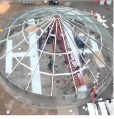
After the first two rings of wall sheets are erected, roof rafters and purlins are all attached, then all bolts are tightened.
