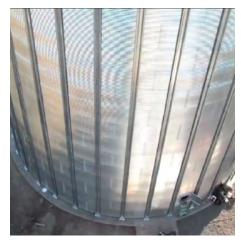
Bottom stiffeners and the bottom stiffener assemblies are installed. Silo is anchored to precast anchor bolts in the foundation.
