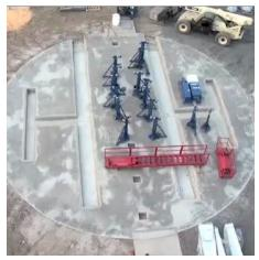
Silo jacks are used for erecting the silo walls.
