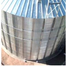
Wind rings can now be bolted to the clips at the stiffeners. Wall sheets continue to be added as silo is jacked up one ring at a time. Additional tiers of stiffeners are added after every two rings.
