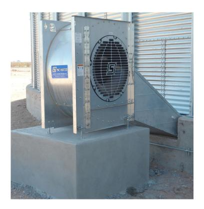
Aeration can control moisture accumulation by creating a uniform grain temperature throughout the grain mass. An effective method is to move small quantities of air (1/10 CFM/bushel [about 6.25 M3/Hour/metric ton]) through the grain more or less continuously until temperatures are equalized to within a range of the average ambient air temperatures. In this regard, the goal is to maintain the grain temperature within 4° to 5°C of the average daily ambient air temperature.
