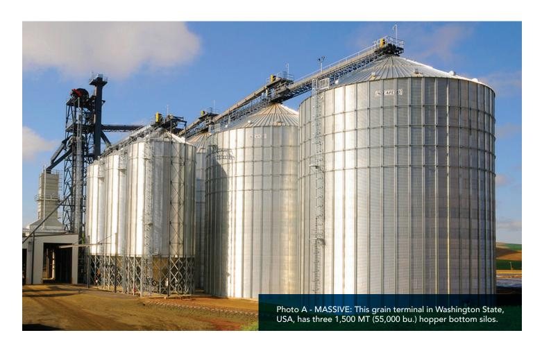
Day silos adjacent to the rice mill also utilize hopper bottom structures because of their ability to discharge the grain using gravity. No expensive sweep augers are required and there is minimal damage to the rice kernels.
