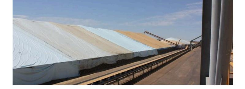
were pre-manufactured to fit the shape of the storage. Usually in the spring time the pile walls were breached and large loaders entered the storage area to fill trucks, taking the grain to feed mills, rail loading facilities, country elevators and export storages.
