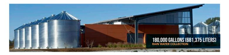
SCAFCO designs and manufactures water tank systems in various diameters with wall heights up to 14 feet (4.27 m) and capacities in excess of 100,000 gallons (395,000 Liters). (Larger tanks available upon request)
